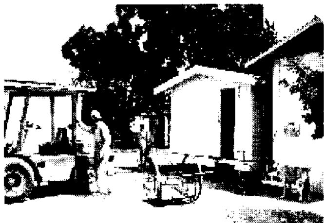
Moving an old building to make room for the new rest room buildings.
