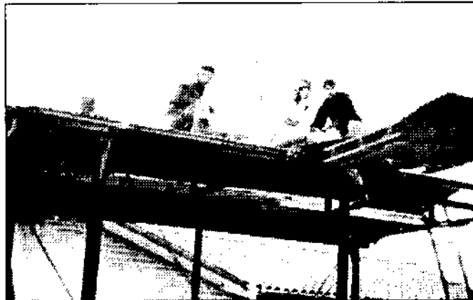
Richard, Will and Aaron Hathaway put the roof on shelter for 1911 Case Steam Tractor. 12/08/93
