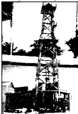
Below: Miniature drilling rig built by J.I. Hathaway in 1928.
